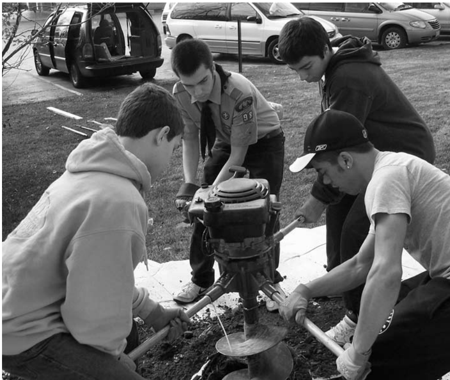
?? and Gerald Gaughan in the background and ?? and ?? in the foreground brace themselves to control a four-man power auger to dig a hole for the post of the new bench.
