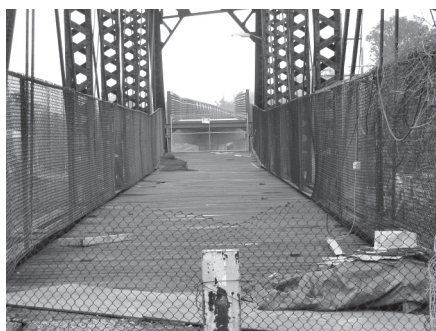
Construction crew reused the old iron truss from Volunteer Bridge in Wheaton for the new bridge. Deck now has a slight grade to it.
