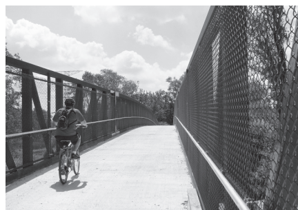
A cyclist rides over the Wayne bridge. Notice how high the railings are. The bridge also has a new type of deck surface that benefits equestrians.
