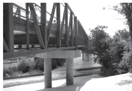
Two column supports hold the new bridge in Wayne, which is between Smith and Army Trail roads.
