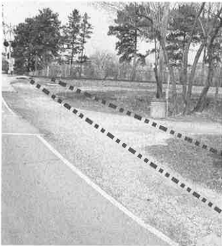
A sidewalk along Chase Street would address safety concerns
