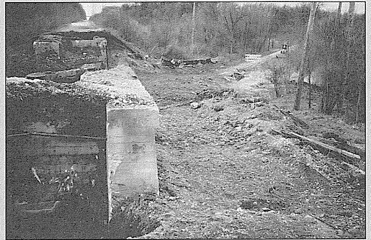
Old Great Western Railroad bridge abutments are uncovered prior to demolition. Illinois Prairie Path heads northwest to Elgin (upper right).
