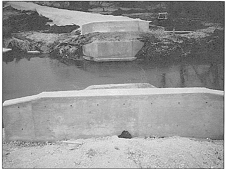
New abutments are ready for installation of bridge across West Branch of DuPage River in Winfield Mounds Forest Preserve. New IPP section heads south to old Chicago, Aurora and Elgin Geneva Spur right-of-way.
