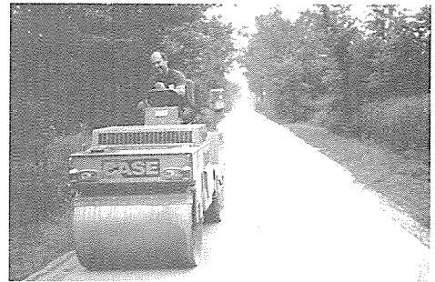
New limestone surface is rolled as smooth as a sheet of paper. Two days later it was already badly dented by horses' hooves.
