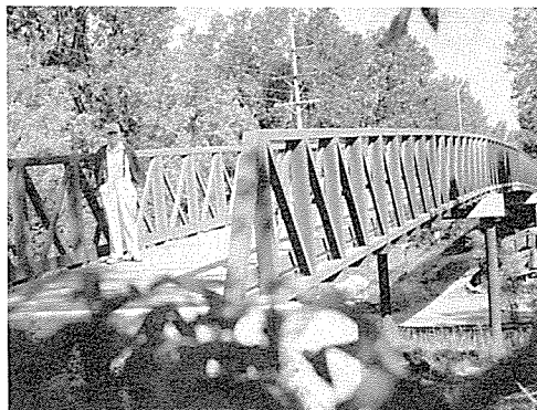
New bridge over Rte. 25 erected by Kane County Forest Preserve District.
