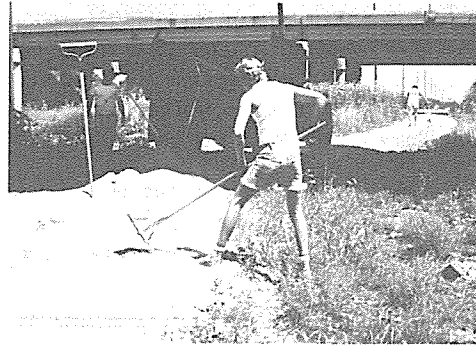
Bob Bain spreads limestone screenings on Path under I-290 bridge, Elmhurst.
