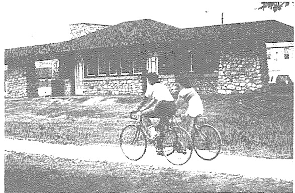
THE RESTORED ARDMORE AVENUE STATION.
