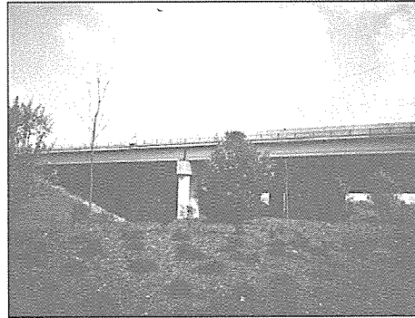
Berm newly planted with trees and shrubs in Berkeley. I-294 overpass in background.
