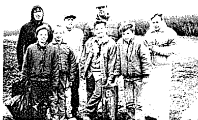
Eagle Candidate Rick Wuollet (second from left, rear) and members of Boy Scout troops 54 and 5 installed RR tie mile markers along IPP Batavia Spur on April 23, a cold day. They also cleaned up the area.
