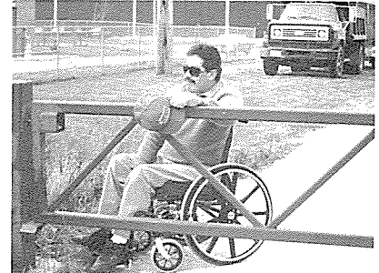
Guerra demonstrates that barrier gate east of Industrial Drive makes access difficult for persons with disabilities.
