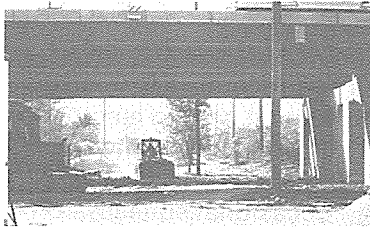
Contractor's front end loader levels trail under I-290 overpass, Elmhurst.
